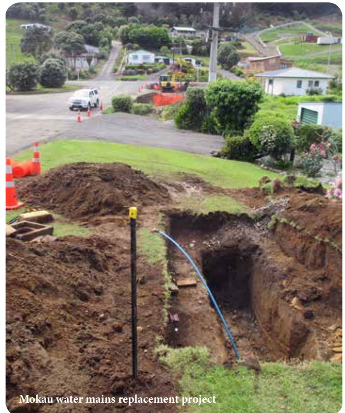
Mokau water mains replacement project
